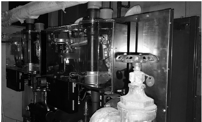
Two of the freestanding boilers are set on a panel, with the other two on the reverse side.
