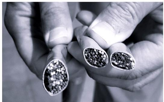
**Three cables with over 200 leads to be spliced back together.**
