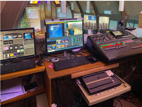
Equipment up in sound booth. From left PC for projection (ProPresenter), PC for video editing (vMix) and also Zoom broadcast, Mixer board for sound Behringer X32, and below control panel for spot lights.
